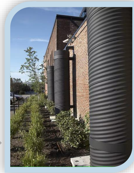
Abb. 6: Retentionszisterne, Quelle: www.archinect.com/firms/project/ 15761943/the-green-building/16356211
